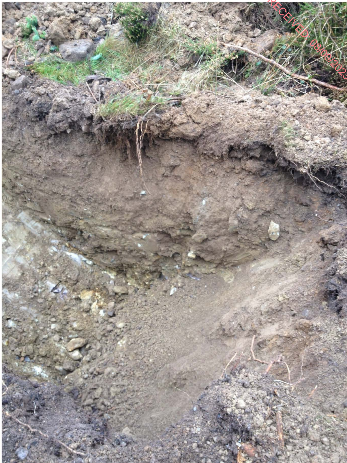
Trial pit at T11
