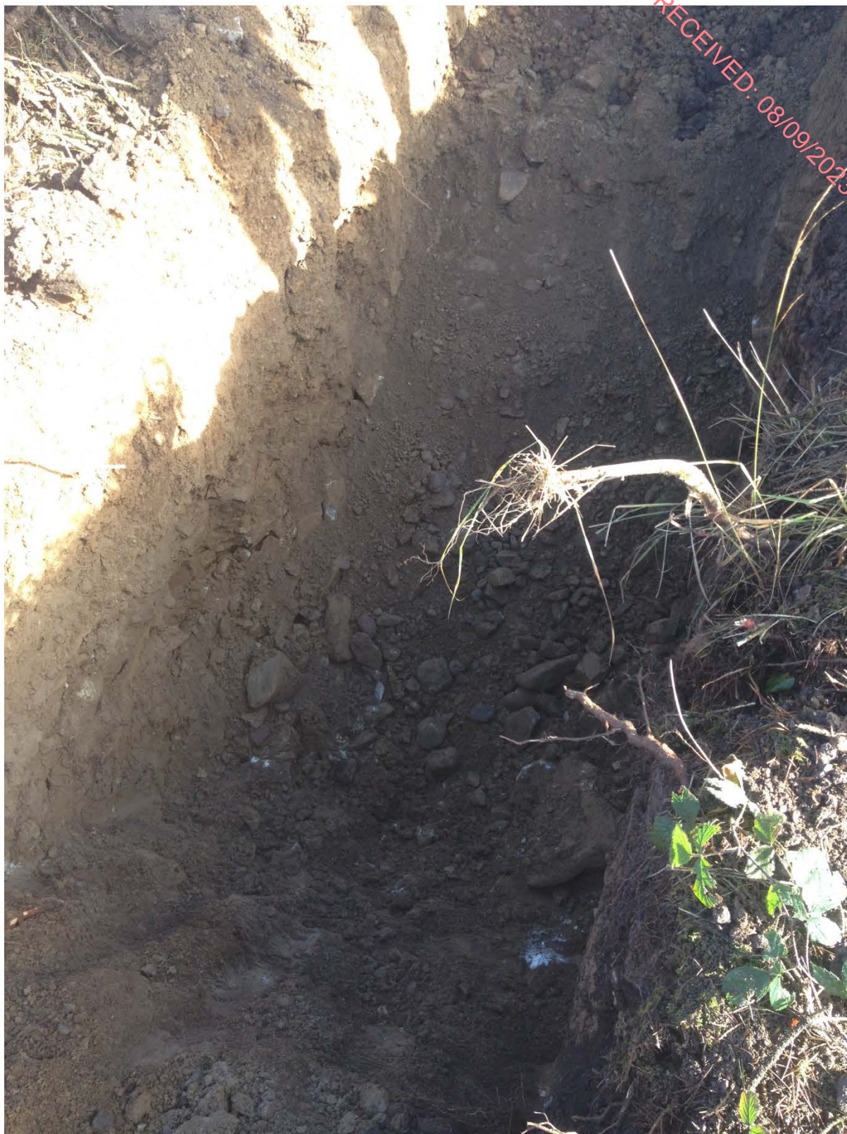
Trial pit at T01
